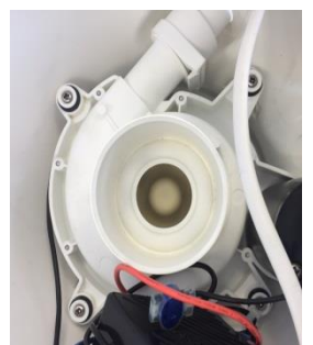
14. Replace waste pump
